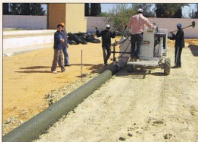
In Libya, CF3000 slipforms garden curb in housing development.
